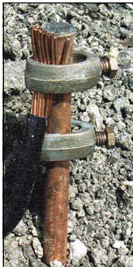
Figure 1. Example - Ground Electrode Installation
